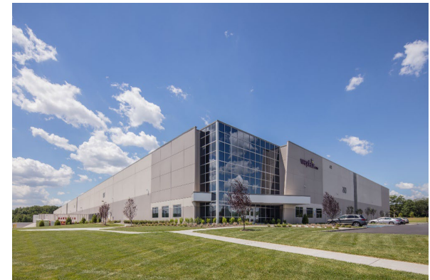
Cranbury Station, Cranbury, NJ
