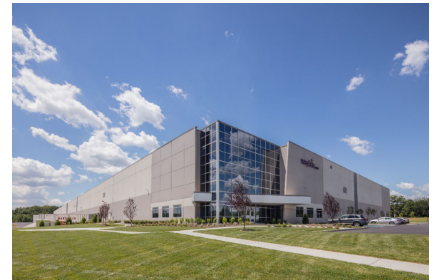
Cranbury Station, Cranbury, NJ
