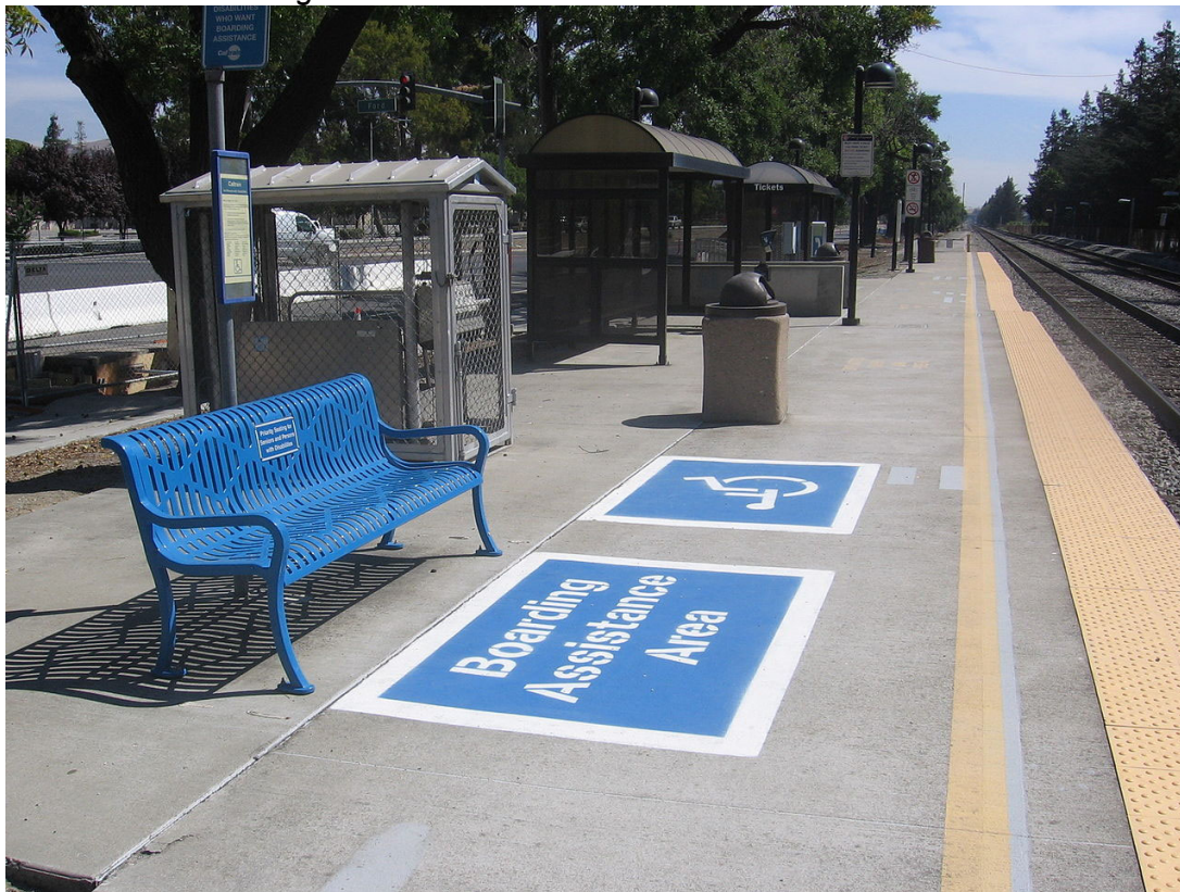
Figure 34: Platform Markings for ADA Access
