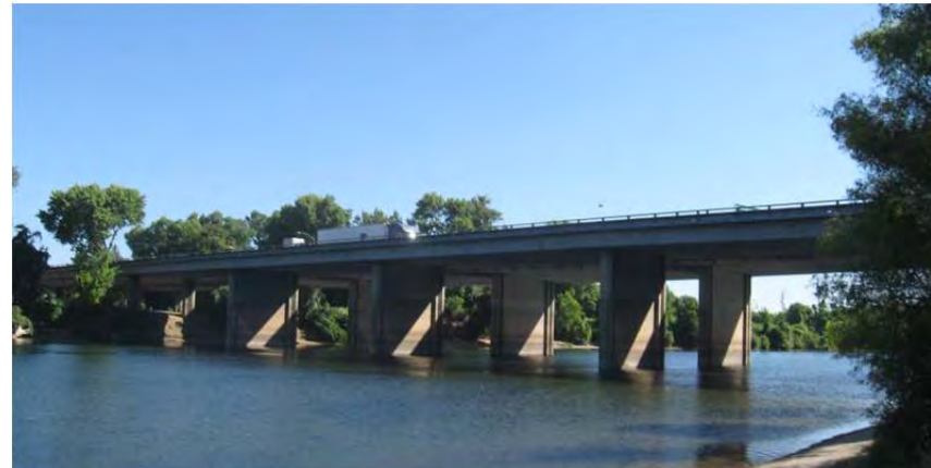
Both the I-5 Viaduct and the Jibboom Street Bridge use piers in the American River
