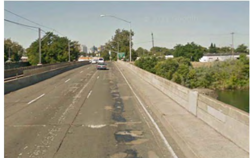
Existing Sidewalk on SB SR 160
